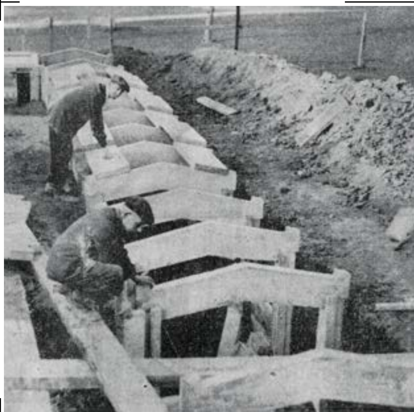
Concrete-lined ARP trenches were constructed in Midsummer Common between Auckland Road and Brunswick School.
